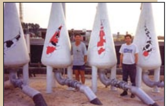
Cones which supersaturate the water with oxygen via pressure.
