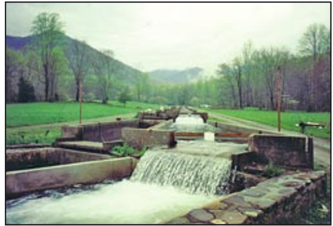
FAR LEFT: Raceway system that picks up oxygen via 18" drops at every section.
